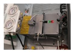
Interlocked three position disconnect switch for isolating and earthing with electric operation
