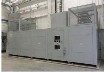
Used as a multiple-step, second-order harmonic filter bank in a large wind-turbine drivetrain facility
