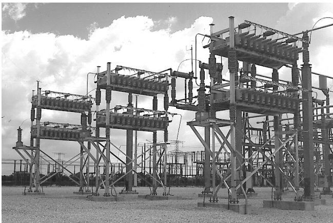
Figure 1. Externally fused capacitor bank
