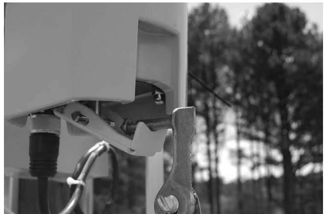
Figure 3. Contact position indicator (switch shown in open position)
