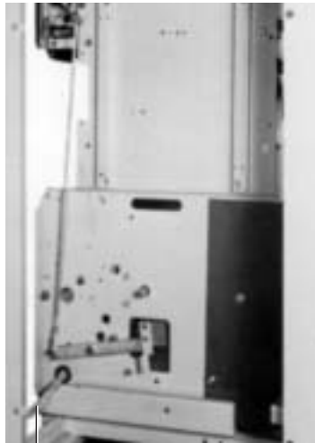
Mechanical Interlock Between Isolation Switch and Contactor Slide-Out Design
