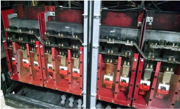
Figure 10. Phase segregation barriers
