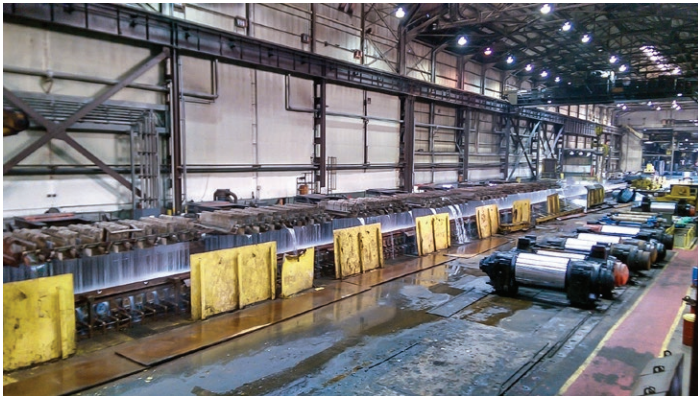
HROT cooling water.
