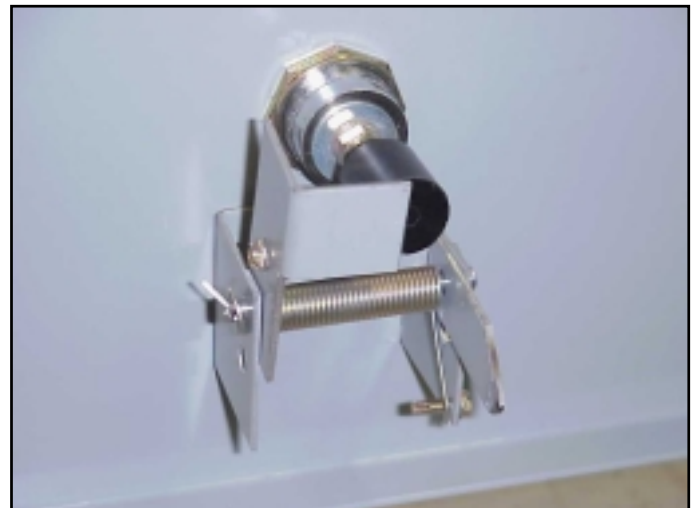
Figure 10: Latch Release Mechanism (Rear of Medium Voltage Door)
