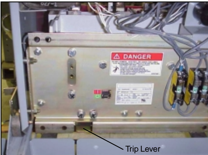
Figure 8: Mechanical Release Lever
