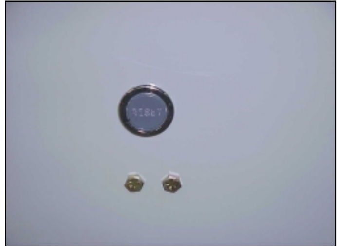
Figure 9: Latch Release Button (Front of Medium Voltage Door)
