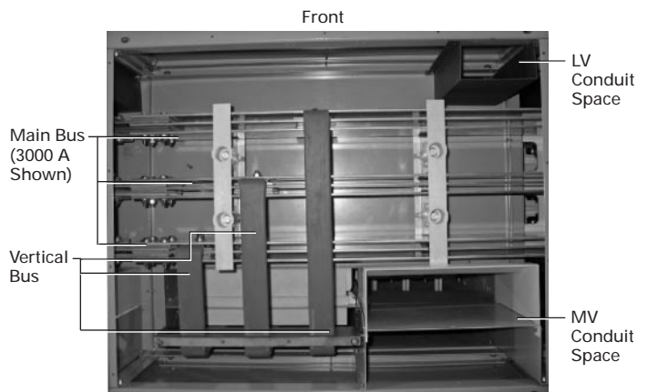
FIGURE 13. MAIN BUS COMPARTMENT, TOP VIEW
