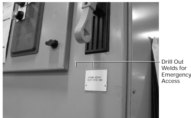
FIGURE 29. DRILL LOCATION FOR EMERGENCY ENTRANCE TO MV COMPARTMENT
