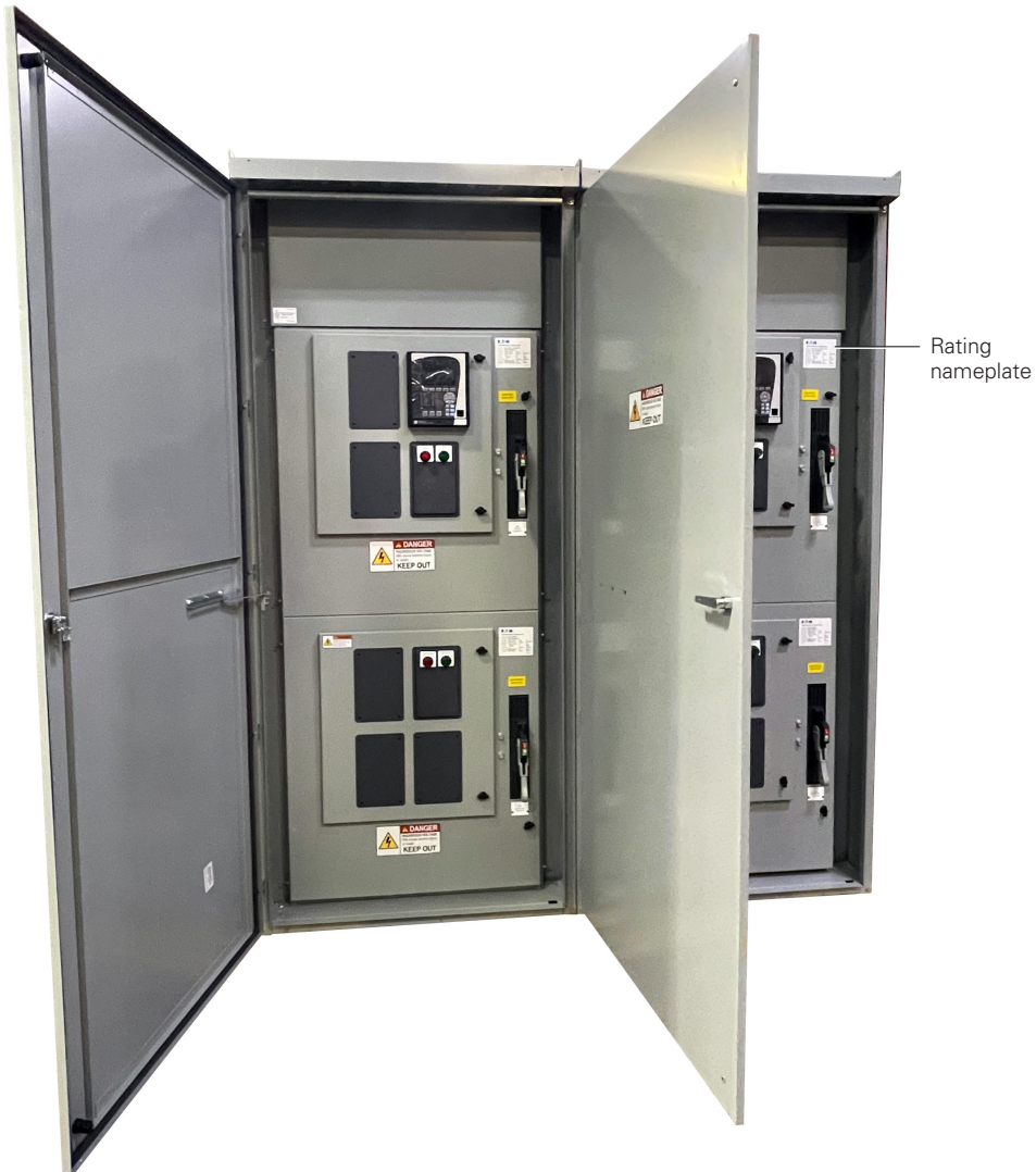
Figure 1. Rating nameplate on the door.
