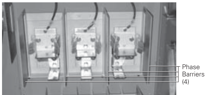
Figure 19. Lower Fuse Mounting with Optional Fuse Clips
