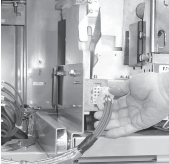
Figure 26. Unplug Control Harness
