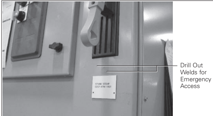
Figure 34. Drill Location for Emergency Entrance to MV Compartment
