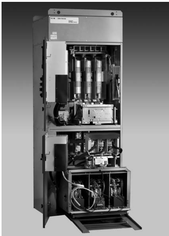
Figure 14. 400A MV4S starter (doors open)
