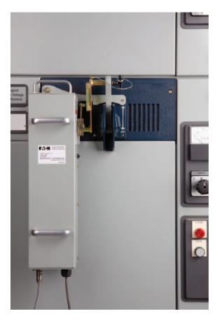
For customers seeking to remain outside the arc flash protection boundary when operating an isolation switch, Eaton is pleased to introduce the Classic Remote Operator (CRO).
