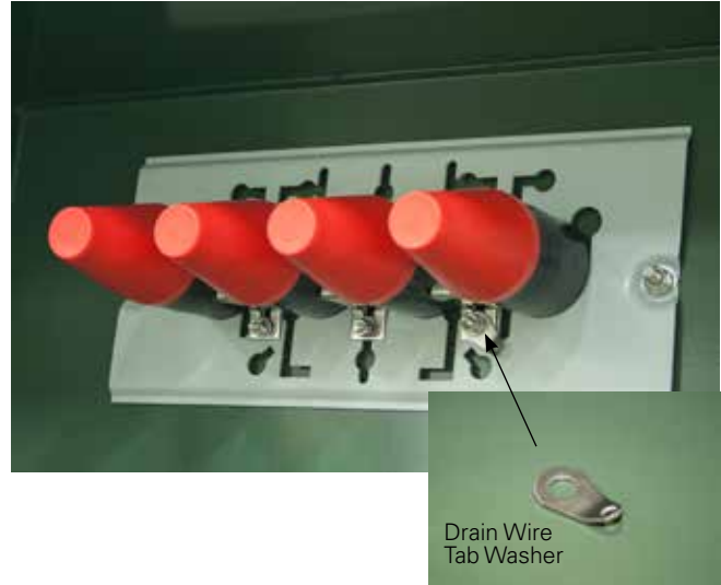
Figure 17. Install drain wire tab washer.
