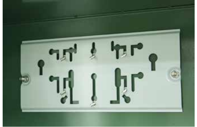
Figure 13. Install carriage bolts.
