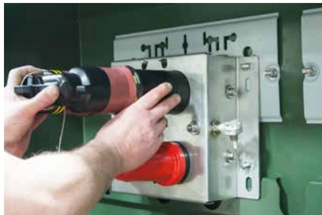
Figure 22. Install Cleer connector on bolts.
