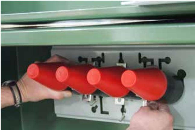
Figure 16. Align u-straps with lower carriage bolts.
