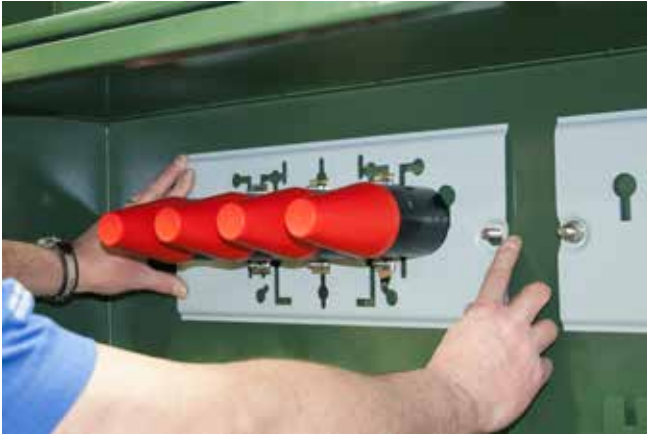
Figure 8. Install mounting plate/junction assembly.
