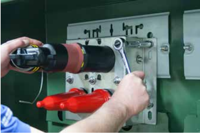
Figure 23. Install hardware and tighten.
