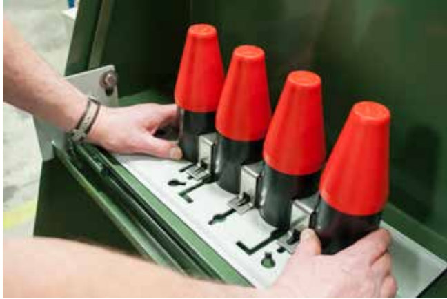
Figure 4. Align u-strap slots with plate slots.
