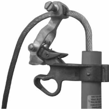
Figure 11. Installing a fuse link in a 200 A fuse holder.
