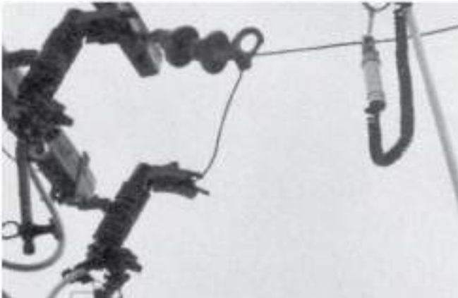
Figure 3. Tool hanging by hotline clamp.
