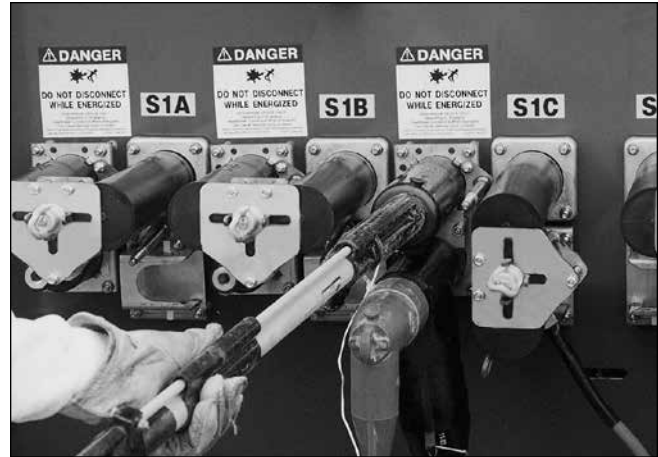
Figure 9. Install U-OP protective cap on exposed bushing.
