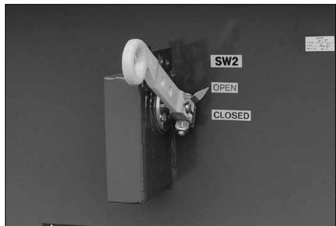
Figure 4. Open switch at both ends of cable.
