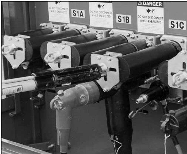
Figure 7. Disengage U-OP operating shaft.
