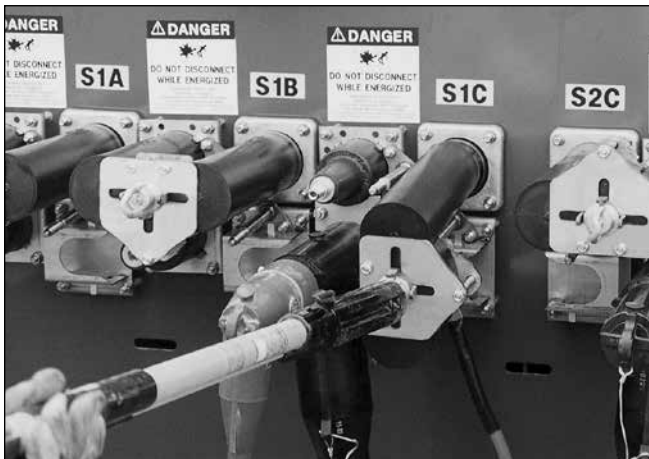
Figure 8. Reorient the U connector.
