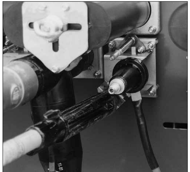
Figure 6. Mount grounded standoff bushing.
