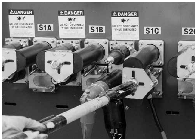
Figure 11. Disengage operating shaft from mating stud.
