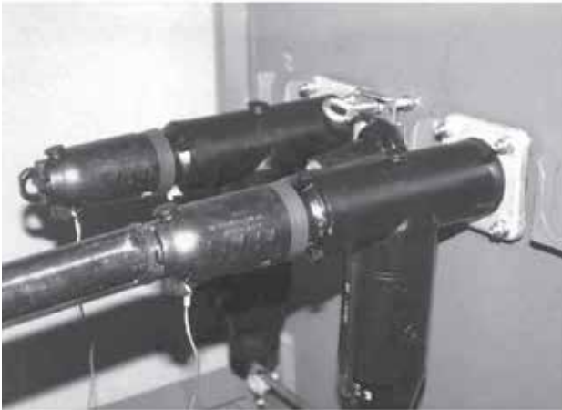
Figure 14. Reinstall 200 a protective cap
