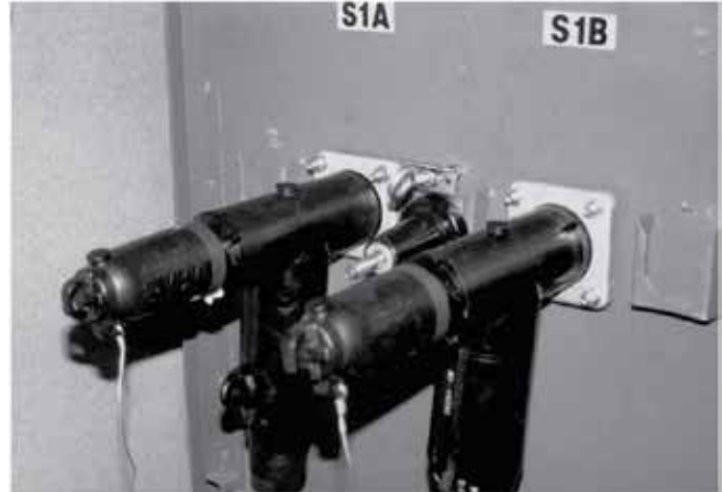
Figure 1. 600 A T-OP II Terminator
