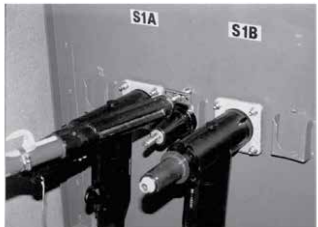
Figure 6. Mount T-OP II standoff bushing
