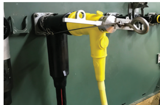
Figure 7. CLEERBAIL and CLEERCHAIN Installation
