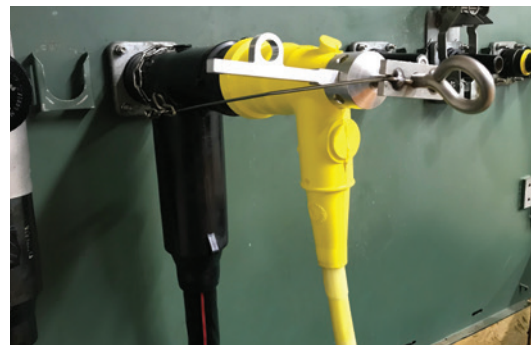
Figure 7. CLEERBAIL and CLEERCHAIN Installation
