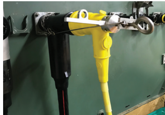
Figure 16. CLEERBAIL and CLEERCHAIN installation
