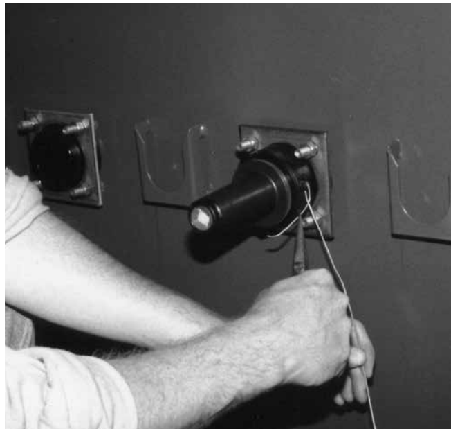
Figure 4. Attach ground lead (15 kV version shown).
