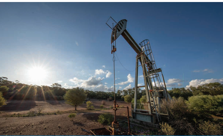
Oil pump stations
