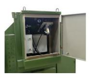
Pad-mounted transformer with VFI and motor operator located in separate compartment for remote open/trip and close capability.
