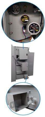
External drain valve with sampler for safer and easier oil sampling.
