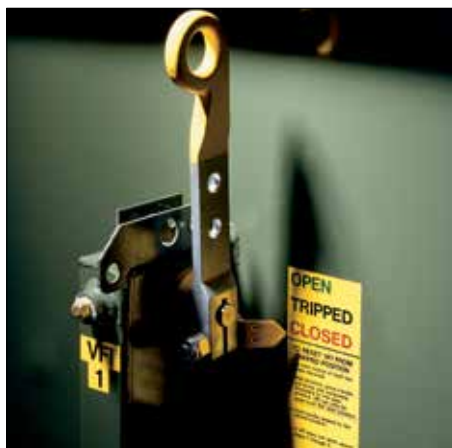
Figure 13. VFI—operating handle.
