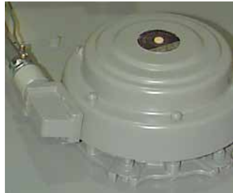
Figure 4. Pressure relief device.
