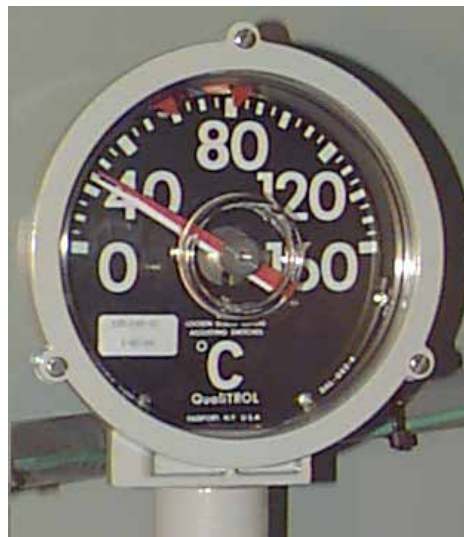
Figure 2. Liquid temperature gauge.
