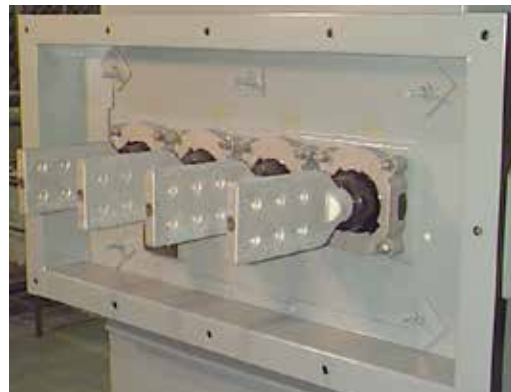
Figure 8. Low voltage bushings.
