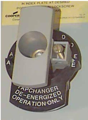
Figure 9. De-energized tap-changer.
