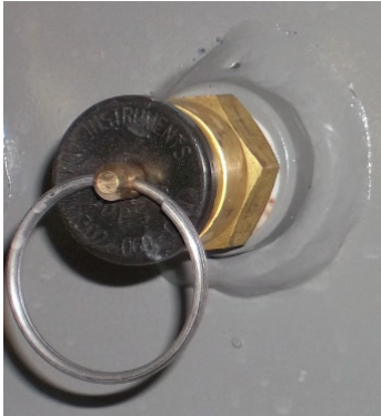
Figure 4. Pull ring on pressure relieve valve to relieve pressure.
