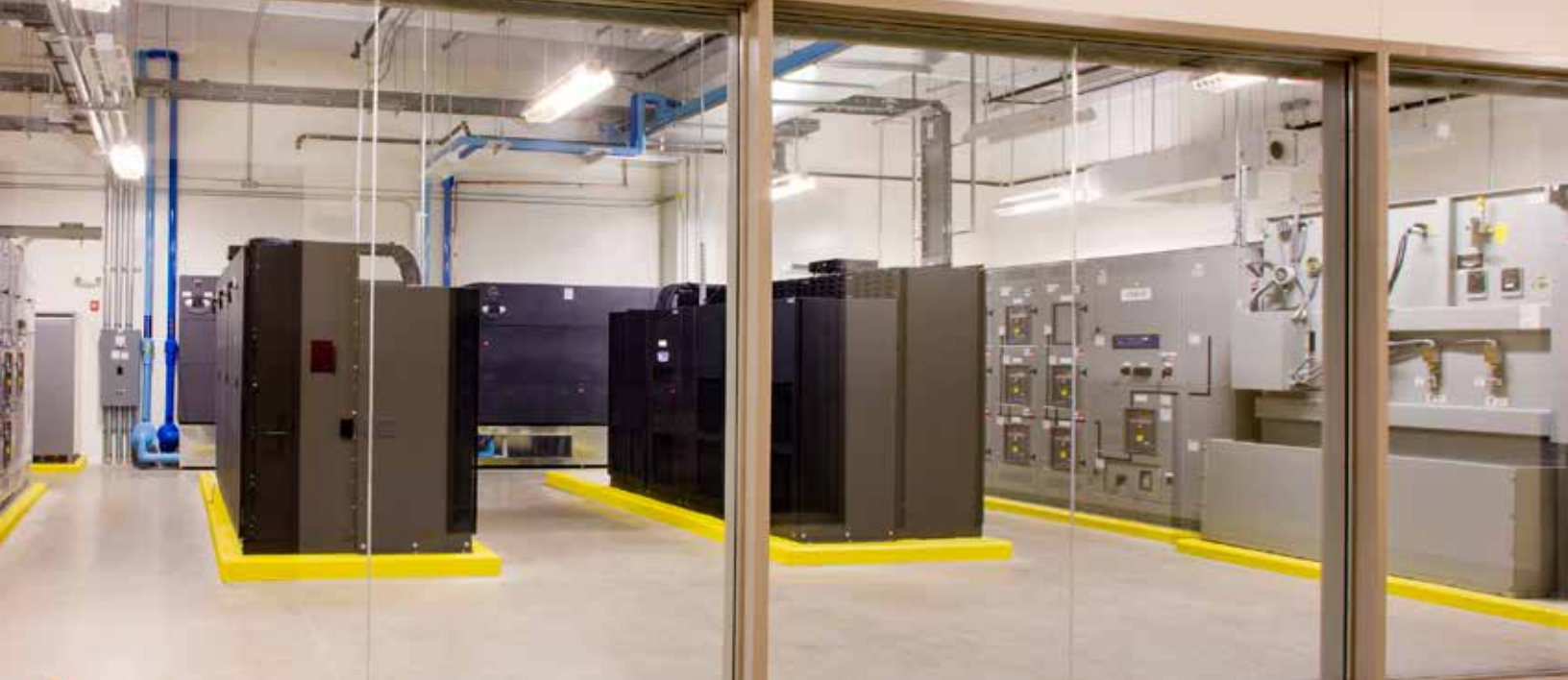
Envirotran™ liquid-filled transformers utilizing Envirotemp™ FR3™ fluid, recognized by the National Electric Code (NEC), Underwriters Laboratories (UL®), and FM Global, have been installed indoors in various applications for more than 15 Years.
