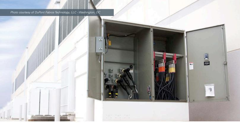
The top priority in critical applications is uninterrupted service. A pad-mounted Envirotran CLT with a tamper-resistant cabinet is ideal for outdoor applications.
