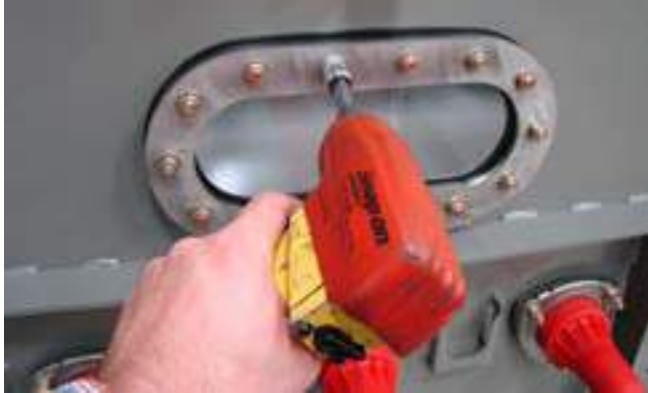
Figure 4. Tighten hardware for visible-break window.
