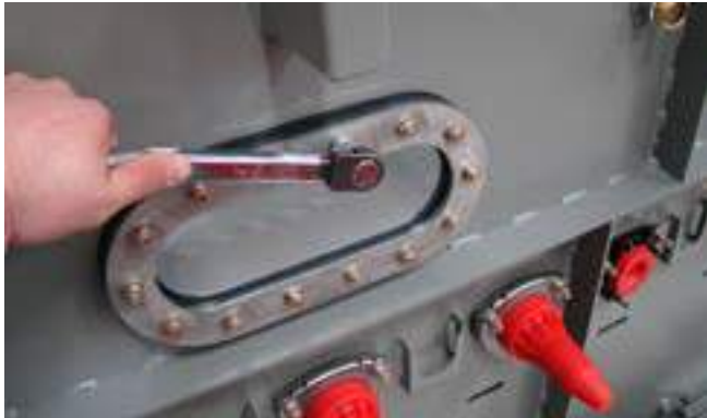
Figure 5. Torque hardware for visible-break window.
