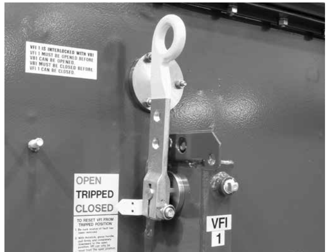
Figure 8. VFI operating handle in the closed position.
