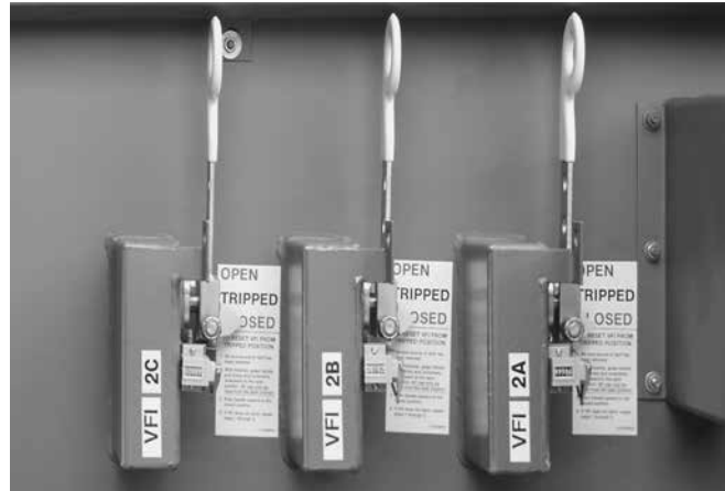
Figure 5. VFI operating handles, single-phase operation.
