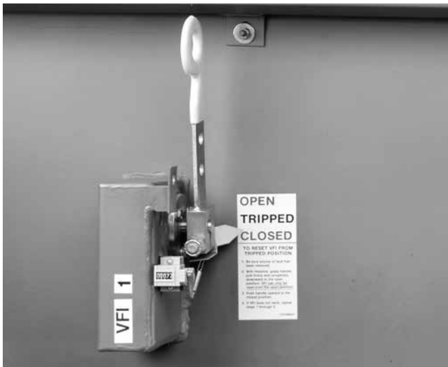
Figure 4. VFI operating handle, three-phase ganged operation.
