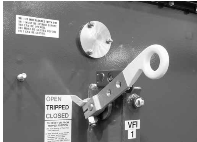
Figure 7. VFI operating handle in the open position.
