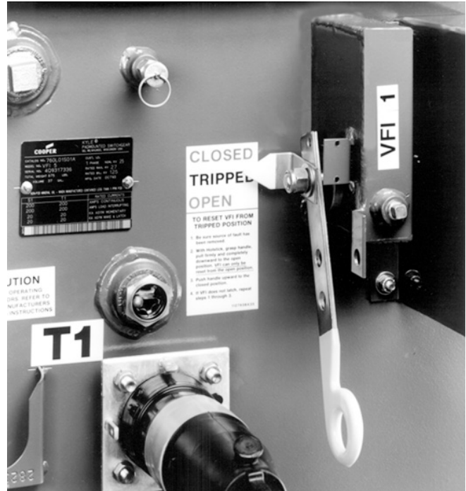
Figure 3. Shrubline VFI operating handle
