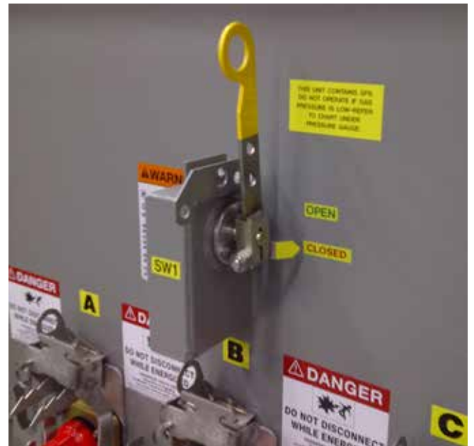
Figure 4. RVAC operating handle.
