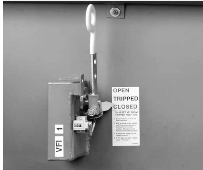
Figure 6. VFI operating handle, three-phase ganged operation
