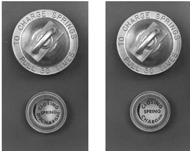
Figure 22. Push-pull charge spring operator indicator before and after manual charging of CI switch
