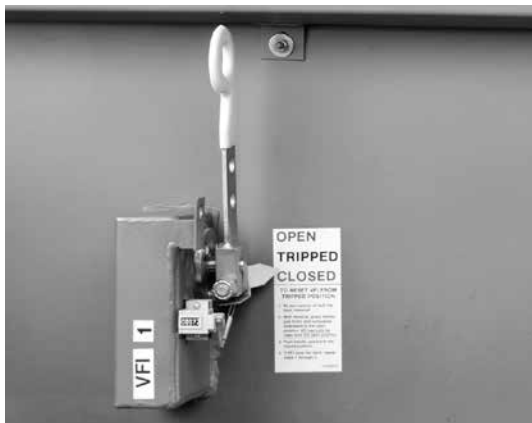
Figure 20. VFI operating handle, three-phase ganged operation
