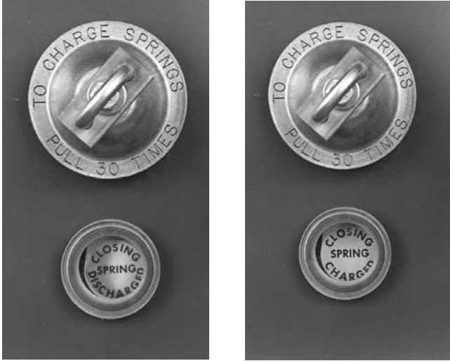
Figure 18. Push-pull charge spring operator indicator before and after manual charging of CI switch
