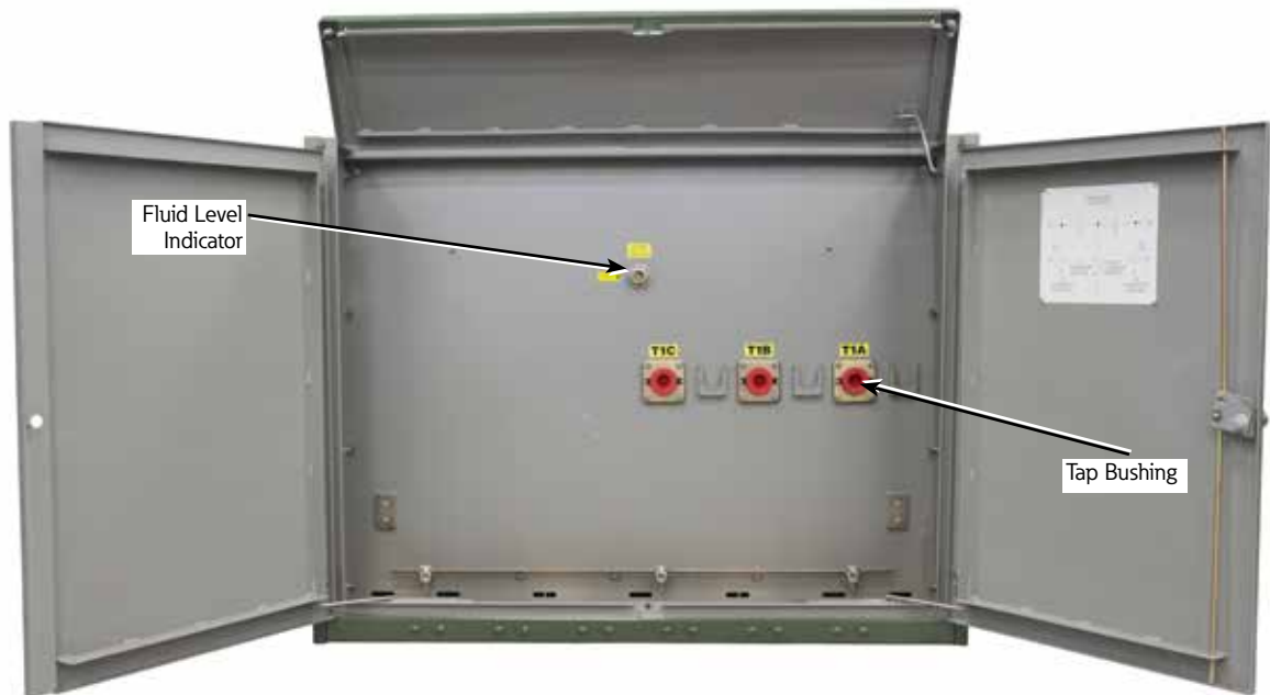
Figure 4. PST Model-6 tap-side features
