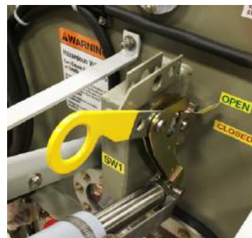
Figure 19. Handle at Open position (pre 2018 units)
