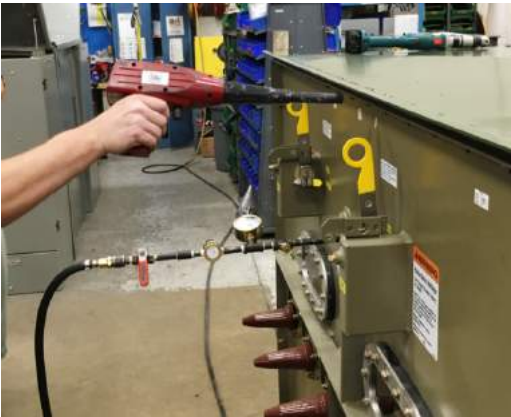
Figure 69. Scanning for leaks
