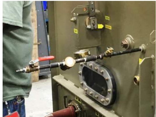
Figure 62. Leak-test assembly installed
