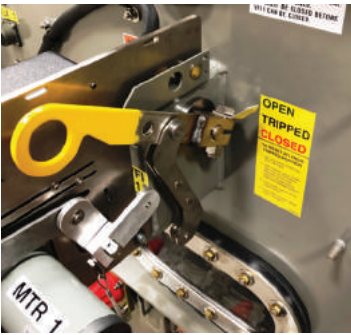
Figure 20. Handle at Open Position (2018 & later)
