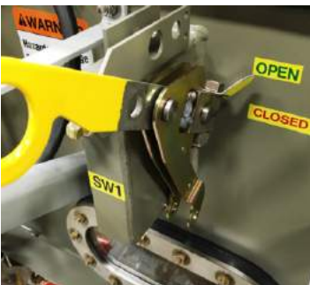
Figure 23. Motor operator removed
