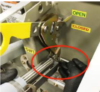
Figure 21. Removing the drive pin (prior to 2018)
