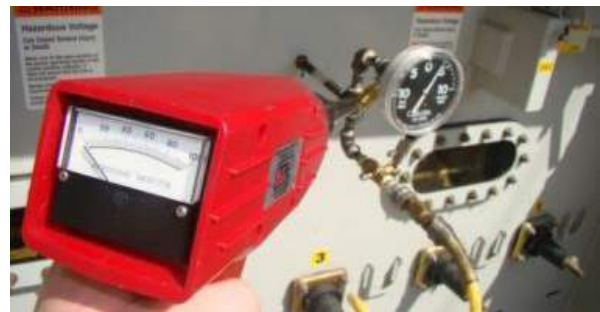
Figure 66. Detector at zero (relief valve closed)
