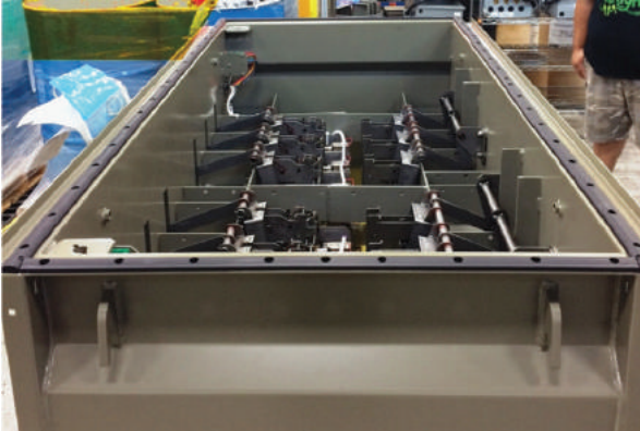
Figure 50. Tamping the fourth (final) gasket
