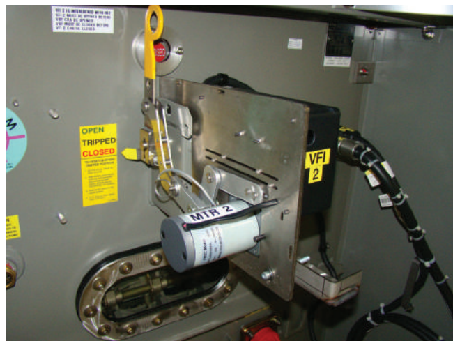
Figure 9. DC Motor actuator - connected
