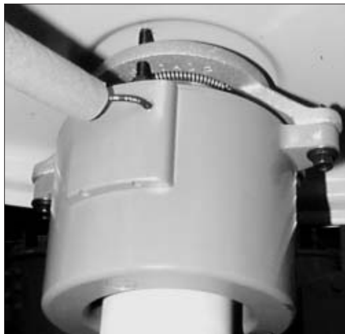
Figure 1-16. Internal bushing mounted current transformer
