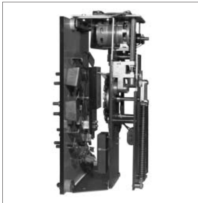
Figure 5-2. 170C Spring-drive Tap Changer
