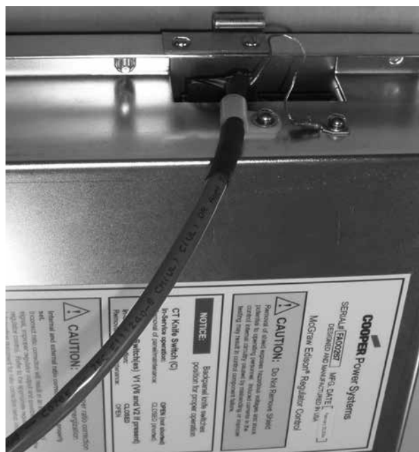
Figure 15. Connecting to the interface cable to the CL-6A control panel
