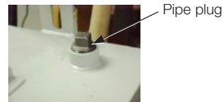
Figure 15. Control box coupling with pipe plug.
