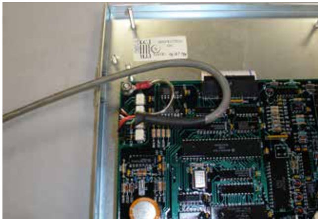
Figure 15. Connecting interface cable to CL-5 control panel.
