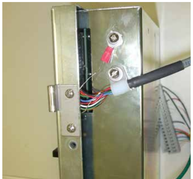
Figure 6. Connecting interface cable to CL-6 control panel.
