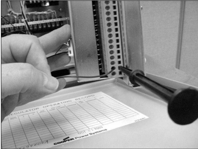
Figure 7. Brown Operational Circuit lead installation.
