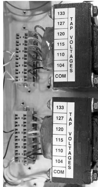
Figure 3-1. Ratio-correcting transformers' connections.
