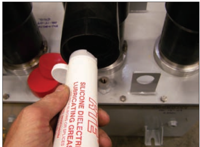
Figure 8. Lubricate housing.
