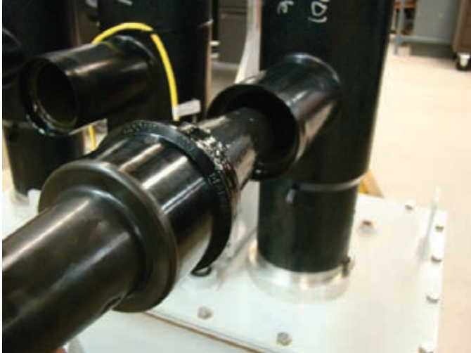
Figure 11. Installation of BLRTP or DCP.
