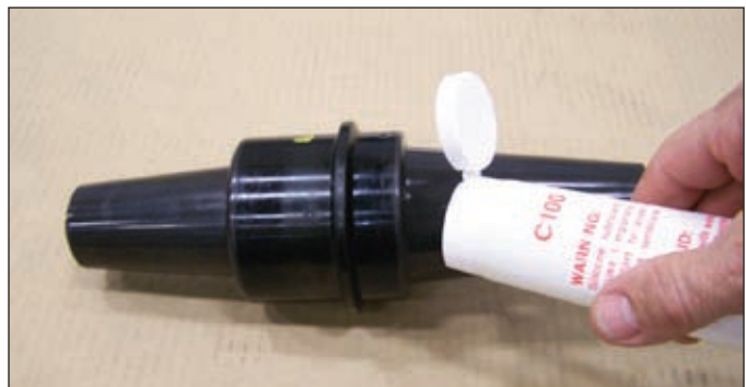
Figure 9. Lubricate interfaces of BLRTP or DCP.
