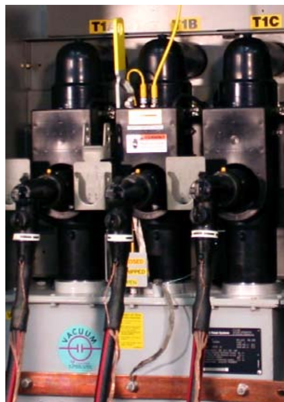
Figure 5. Three-phase ganged operation, vacuum interrupter module.
