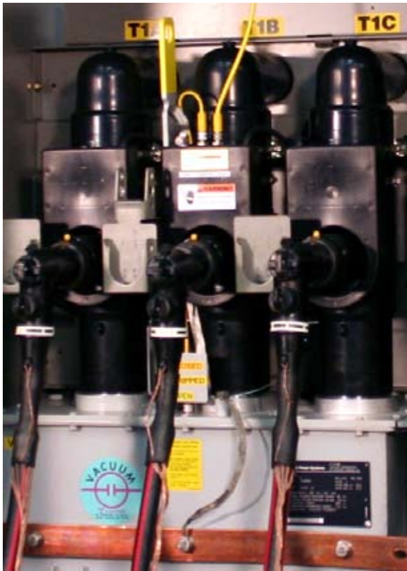
Figure 2. Vacuum interrupter.
