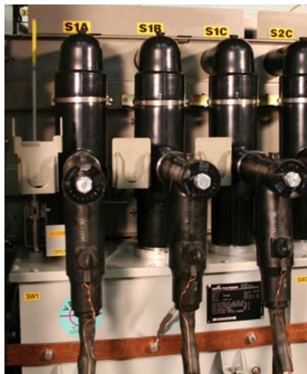
Figure 4. Three-phase ganged operation, load-break switch module.
