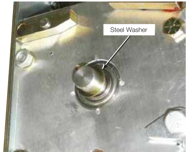
Figure 34. Removing shaft and washer.
