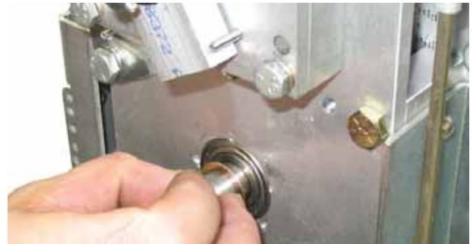
Figure 35. Installing new steel washer from kit.
