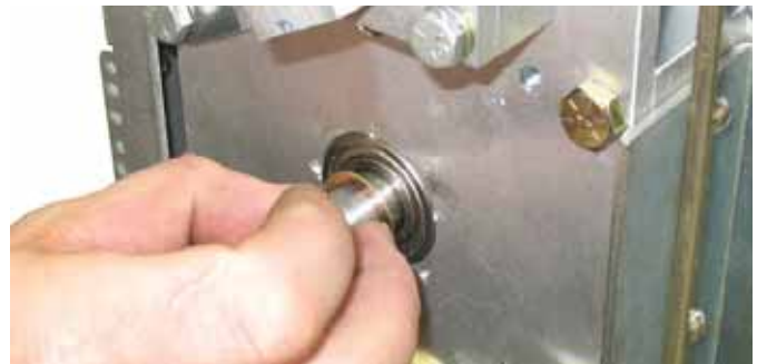
Figure 13. Installing new steel washer from kit.
