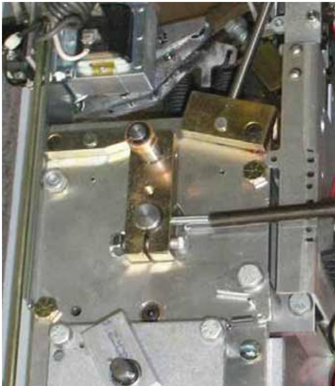
Figure 37. Installing new crank lever on shaft.
