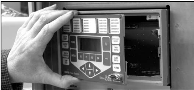
Figure 23. Opening of front panel in preparation of inserting new inserts.
