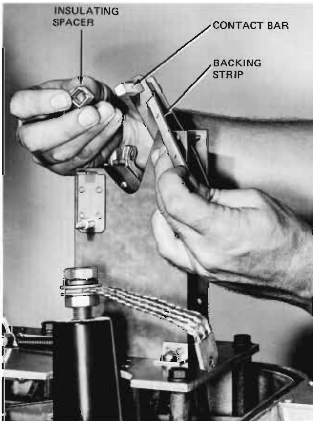
Figure 11 Removing moving contact.
